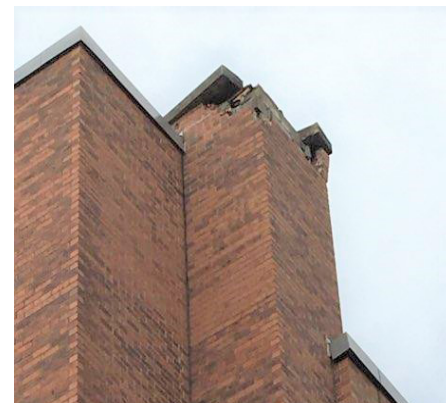
A lightning strike hit not only our chimney stack, but also traveled through the building, damaging a number of our electrical systems.
