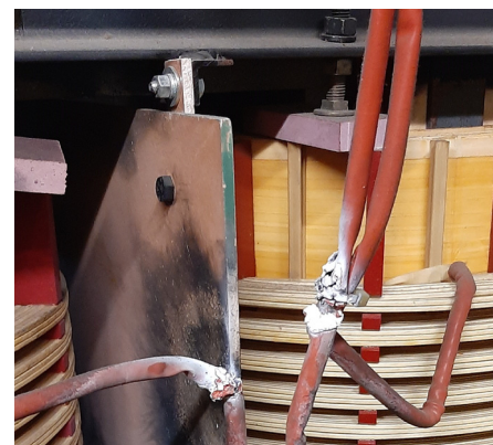
Our electrical transformers were damaged beyond repair. Luckily, temporary ones were put into service until new ones can be installed.
